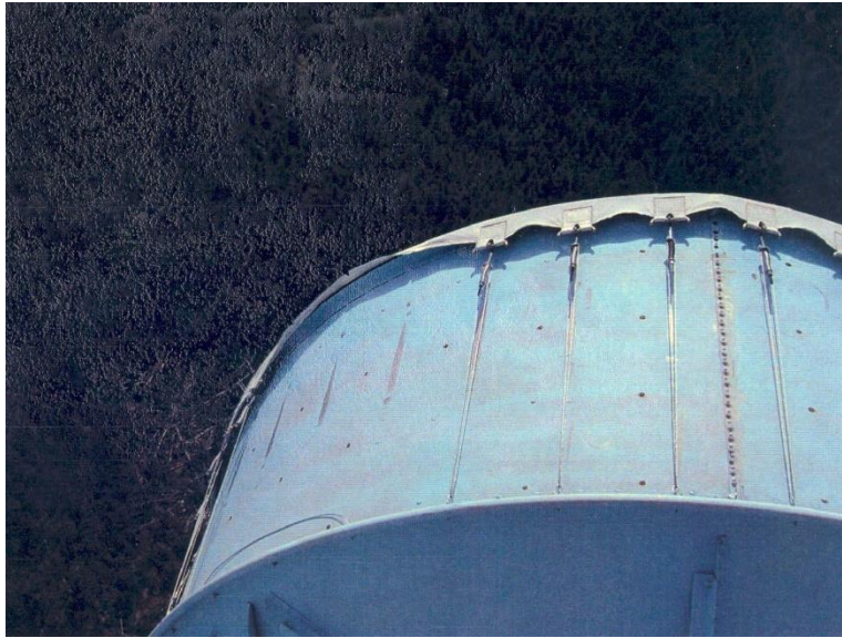
Figure 4: Missing Radome Mounts
