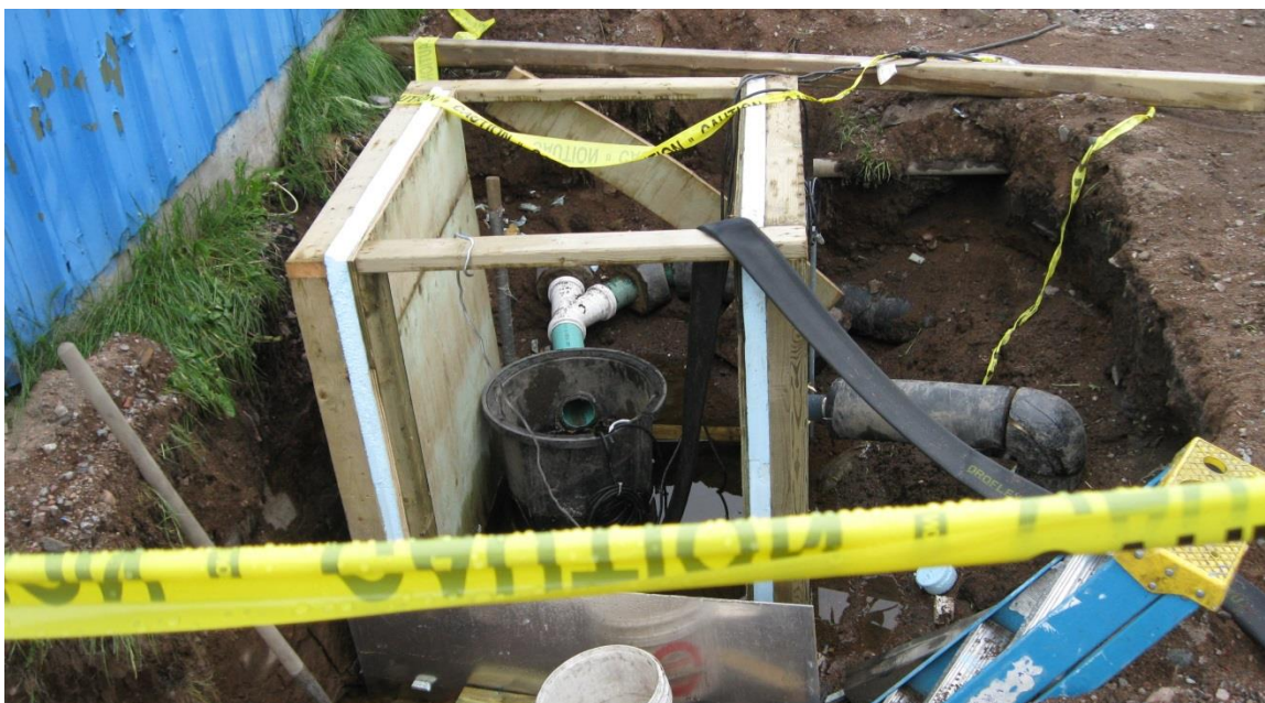
Figure 1: Existing Sewage Lift System
