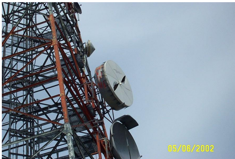
Figure 3: Heavily Damaged Radome
